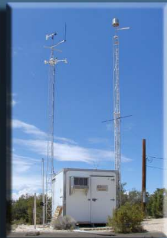
The Abyss air quality monitoring site, located near Hopi Point, is the center for collecting meteorological, ozone, sulfur dioxide, and wet/dry deposition data.
