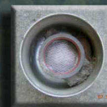
Old inlets became clogged with insect debris.
