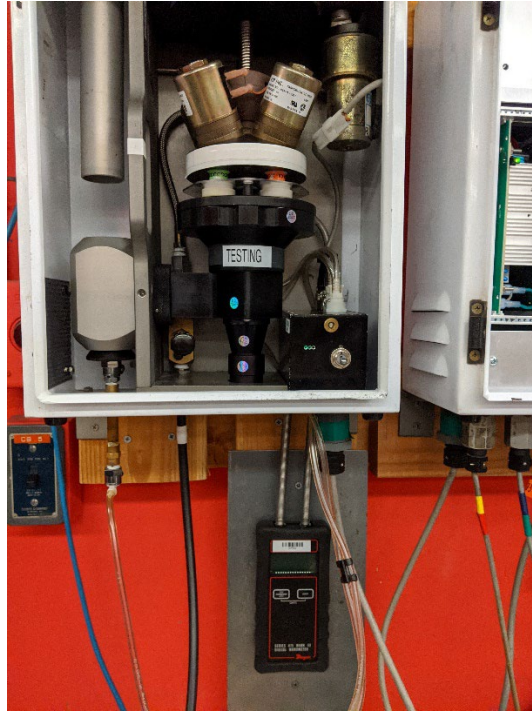
Figure 6. Calibration system with magnehelic flow meter.
